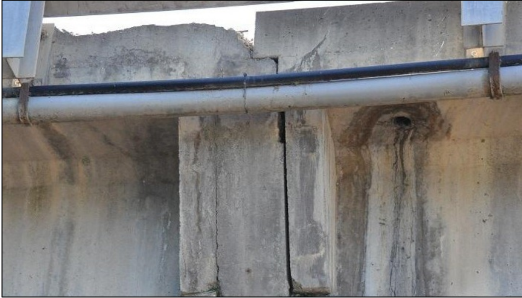
PHOTO 23: BROKEN CONCRETE, EXPOSED RUSTING REBAR, AND WOODEN SHIM (UNDER EAST SPAN)
