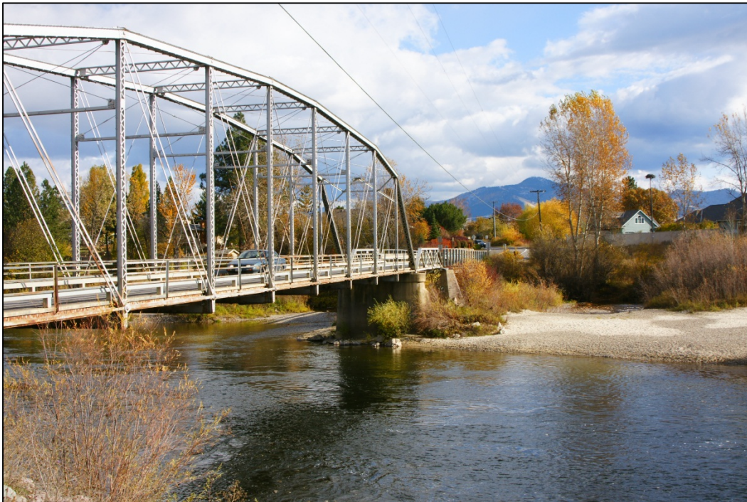
PHOTO 4: LOOKING NORTHEAST – UPSTREAM FACE OF EXISTING BRIDGE
