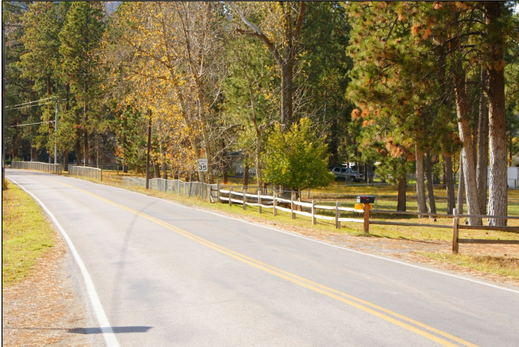
PHOTO 1: LOOKING SOUTHWEST - RIVER PINES ROAD (NOTE POSTED SPEED LIMIT OF 35 MPH)
