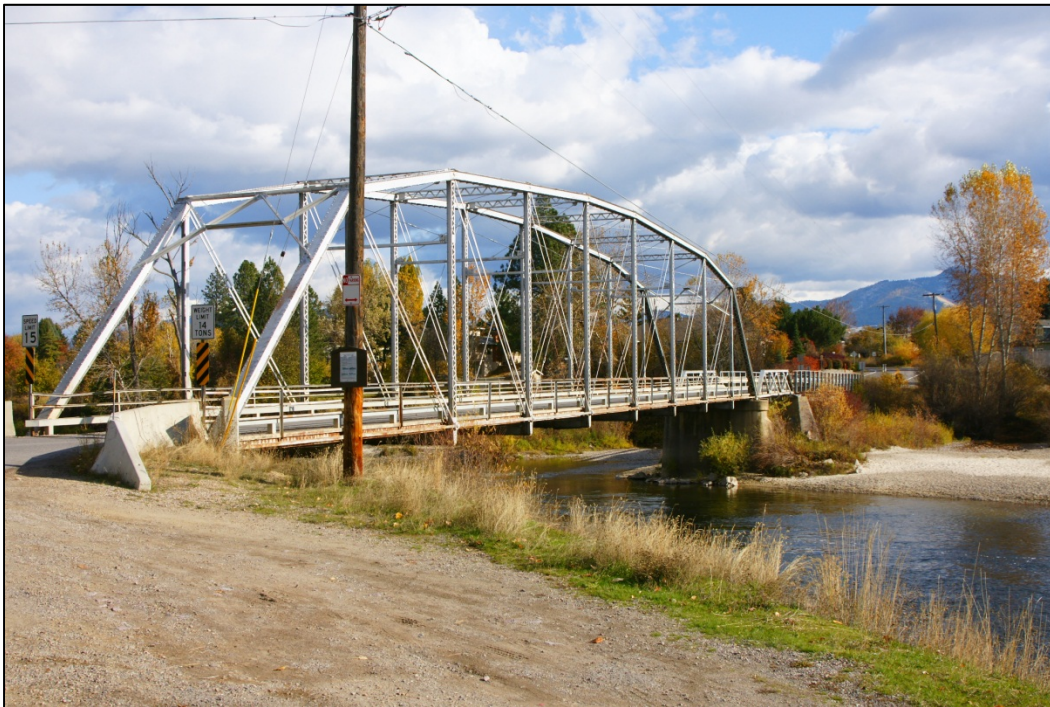
PHOTO 2: LOOKING NORTHEAST – UPSTREAM FACE OF EXISTING BRIDGE
