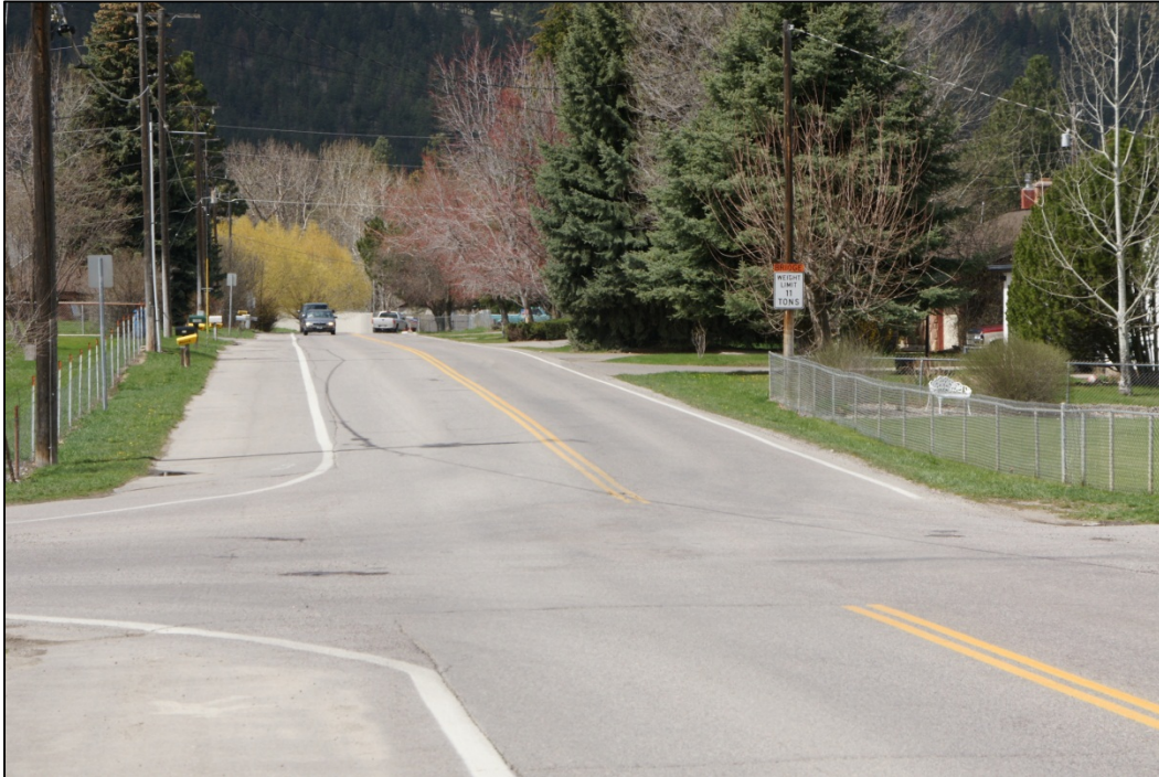
PHOTO 19: LOOKING WEST THROUGH THE INTERSECTION OF NORTH AVENUE AND HUMBLE ROAD
