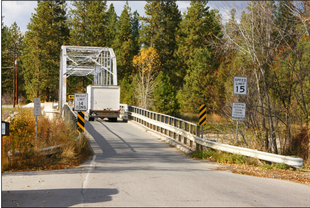
PHOTO 11: LOOKING NORTHWEST ON ALIGNMENT AS TRUCK TRAVERSES EXISTING BRIDGE – 14 TON POSTED WEIGHT LIMIT WAS REDUCED TO 11 TONS AFTER THIS IMAGE WAS TAKEN
