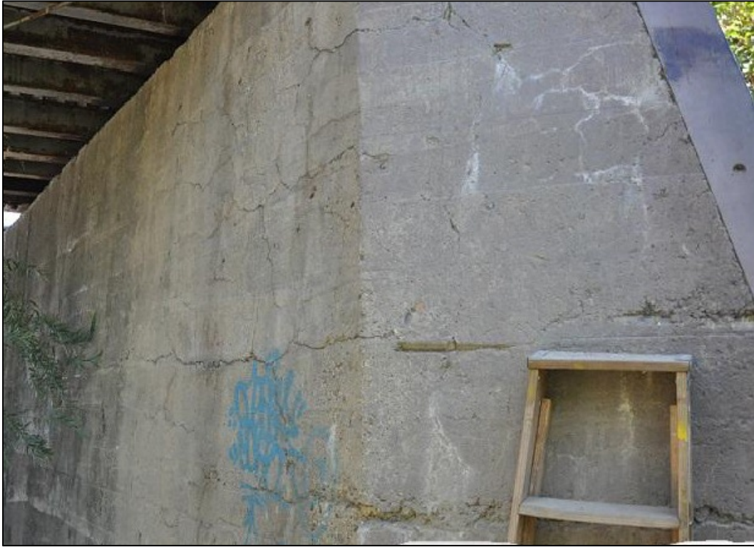
PHOTO 25: CRACKS IN CONCRETE PIER
