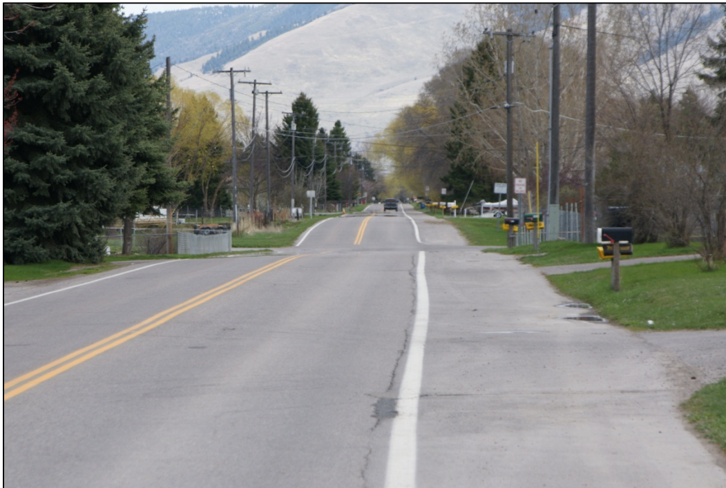
PHOTO 15: LOOKING EAST ALONG NORTH AVENUE – NOTE WIDE SHOULDER ON SOUTH SIDE (RIGHT) FOR PEDESTRIANS/BICYCLES
