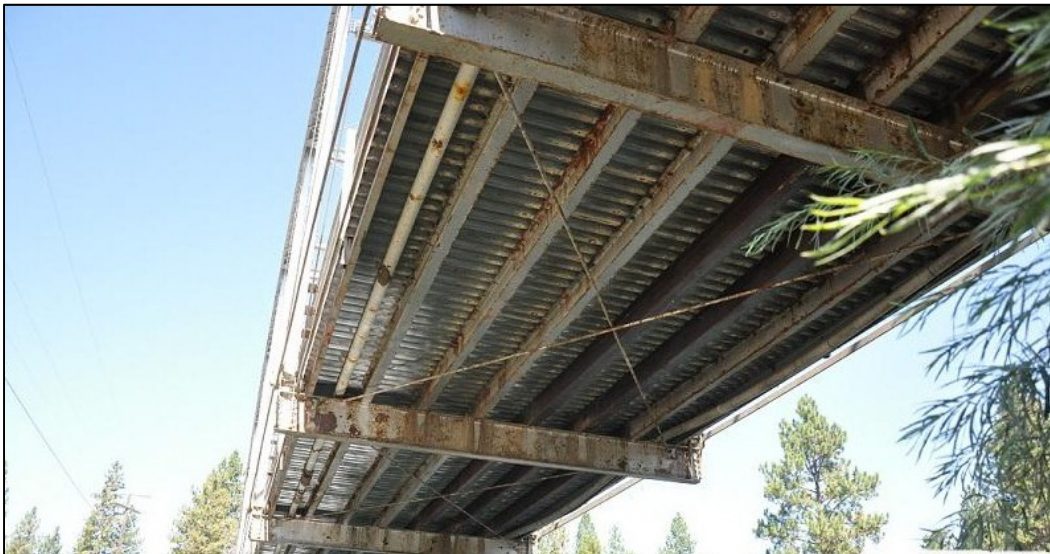
PHOTO 28: STEEL MEMBERS OF VARYING AGES AND CONDITION
