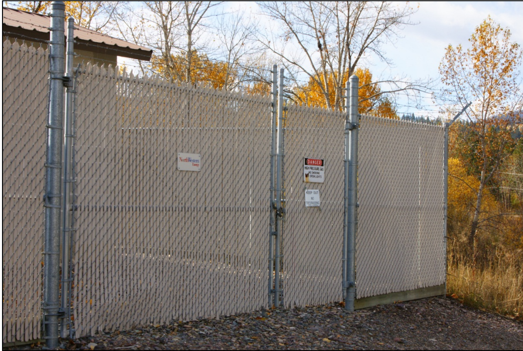
PHOTO 9: NORTHWESTERN ENERGY NATURAL GAS SUBSTATION – ON SOUTH SIDE OF NORTH AVENUE JUST BEFORE CROSSING EXISTING BRIDGE
