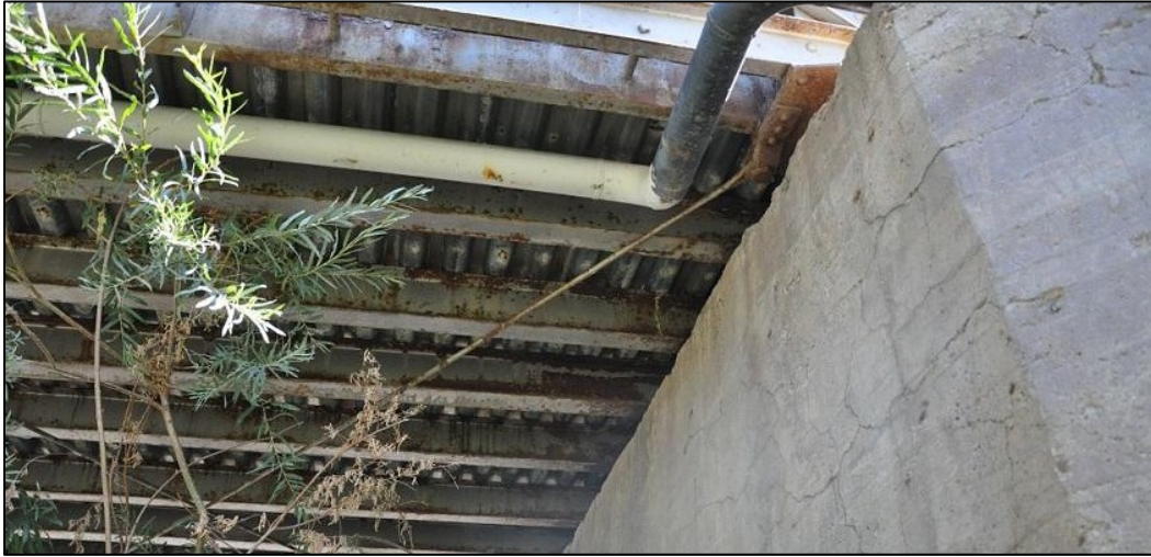
PHOTO 27: RUST ON STEEL MEMBERS (UNDER THE BRIDGE)
