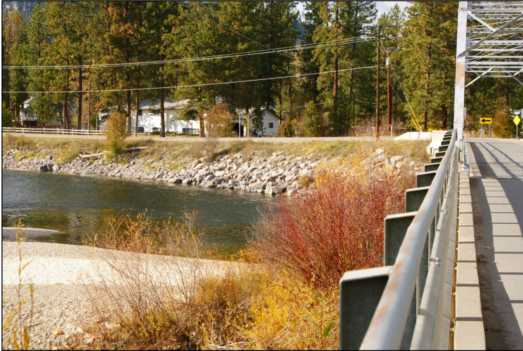
PHOTO 7: LOOKING WEST – NOTE RIPRAP ARMORED FILL SLOPE ON RIVER PINES ROAD
