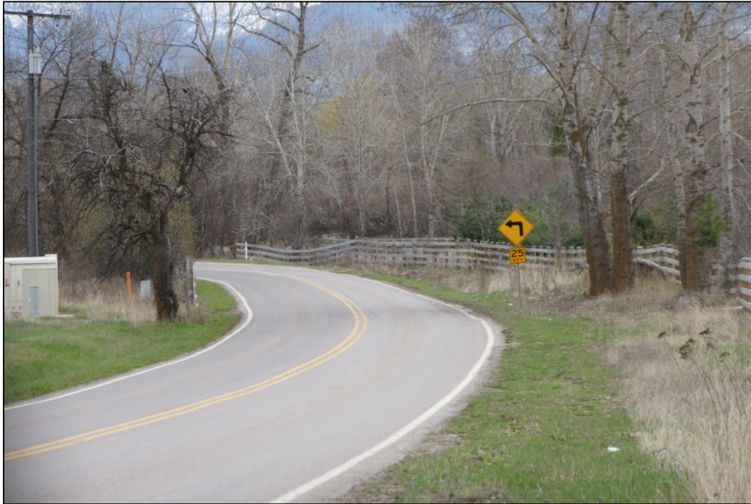
PHOTO 12: LOOKING EAST ON RIVER PINES ROAD AT HORIZONTAL CURVE
