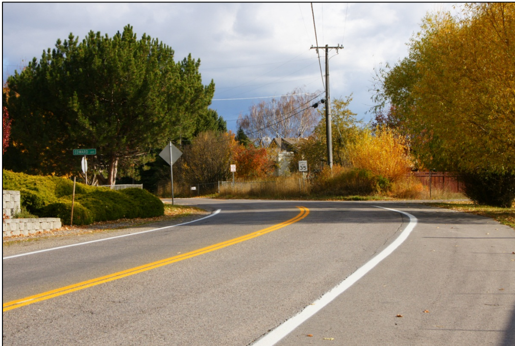
PHOTO 5: LOOKING SOUTHEAST ON NORTH AVENUE – AFTER CROSSING THE EXISTING BRIDGE
