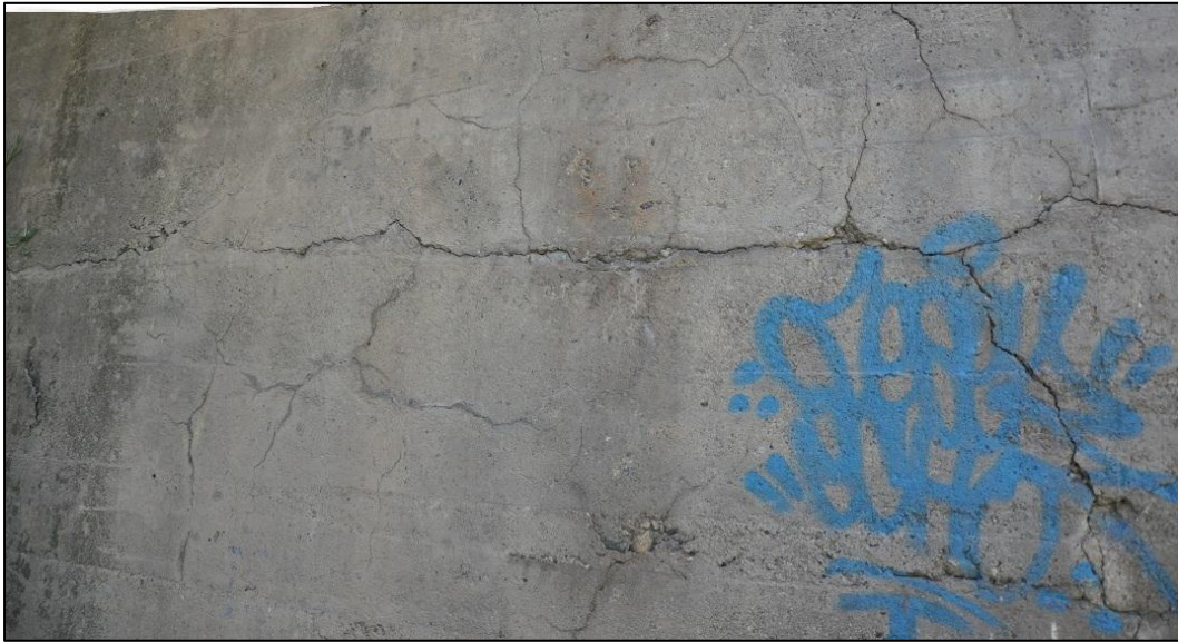
PHOTO 26: CLOSE UP OF CRACKS IN CONCRETE PIER
