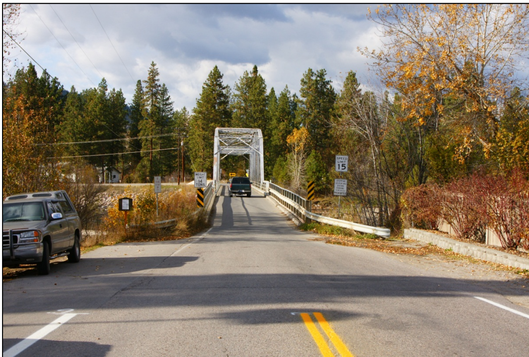
PHOTO 6: LOOKING NORTHWEST ON ALIGNMENT – 14 TON POSTED WEIGHT LIMIT WAS REDUCED TO 11 TONS AFTER THIS IMAGE WAS TAKEN
