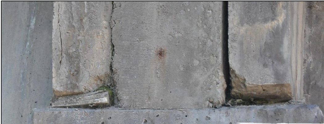
PHOTO 24: WOODEN SHIM UNDER CONCRETE SPAN
