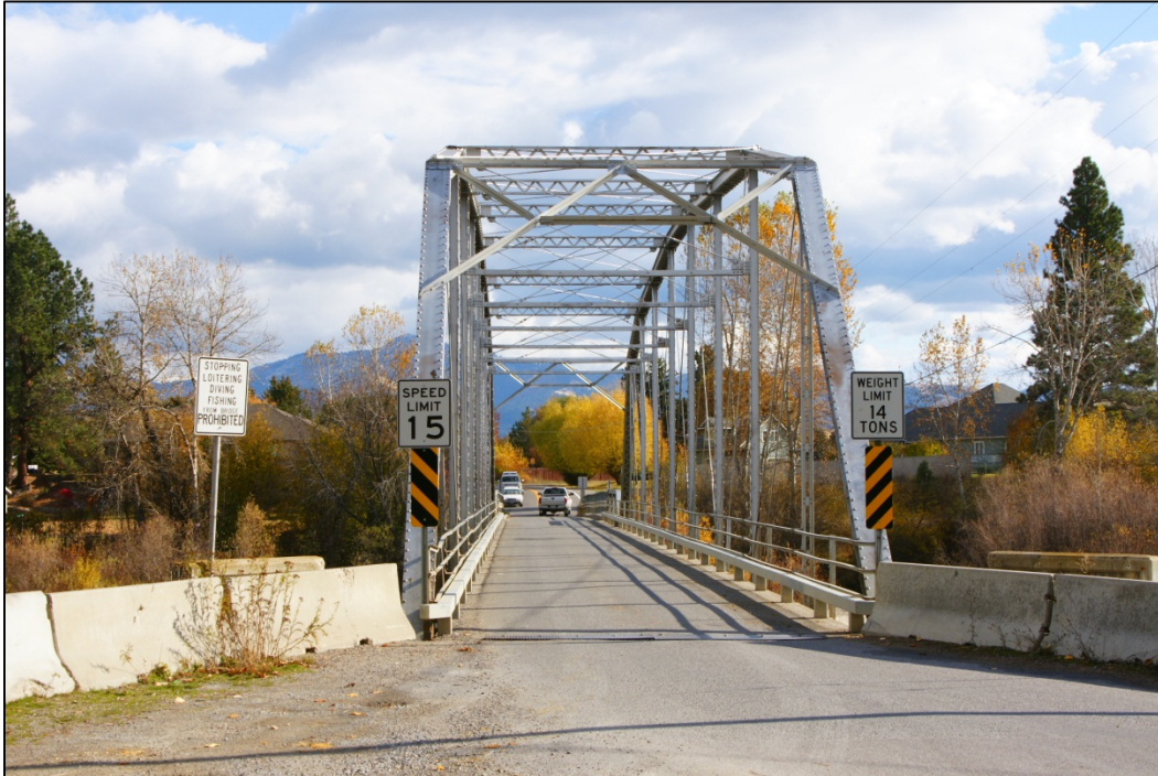
PHOTO 3: LOOKING SOUTHEAST ON ALIGNMENT – 14 TON POSTED WEIGHT LIMIT WAS REDUCED TO 11 TONS AFTER THIS IMAGE WAS TAKEN
