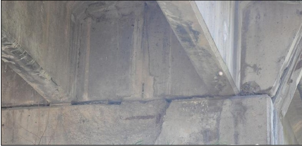
PHOTO 21: EXPOSED RUSTED REBAR AND CONCRETE SPALLING (ON EAST BRIDGE ABUTMENT)
