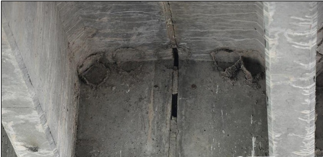
PHOTO 22: MISSING GROUT AND SKEWED JOINT (EAST BRIDGE SPAN)
