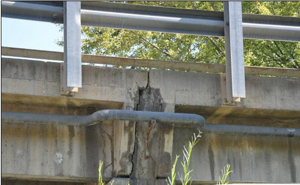
PHOTO 20: DEGRADED JOINT BETWEEN TWO CONCRETE SPANS (NOTE HIGH PRESSURE NATURAL GAS LINE)
