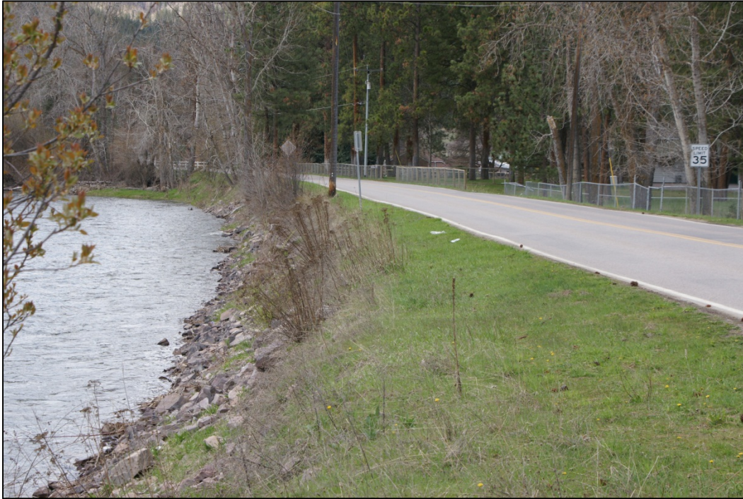
PHOTO 13: LOOKING SOUTHWEST ALONG RIVER PINES ROAD – NOTE RIPRAP ARMORING ALONG FILL SLOPE AND POWER POLE NEXT TO ROADWAY
