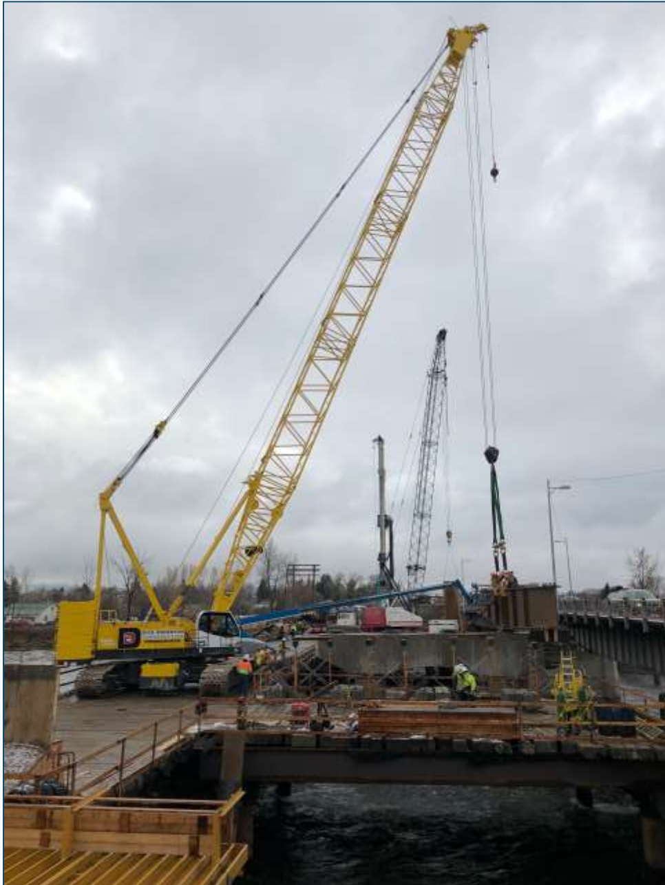
Girder installation on Russell Street Bridge
