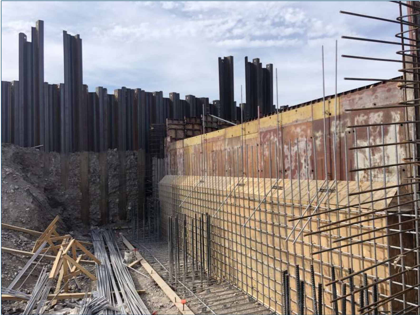
South bridge abutment formwork
