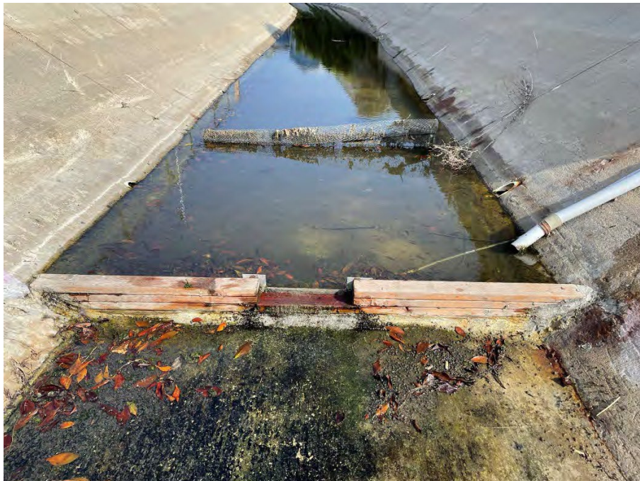
Figure 4-3. Rectangular Weir
