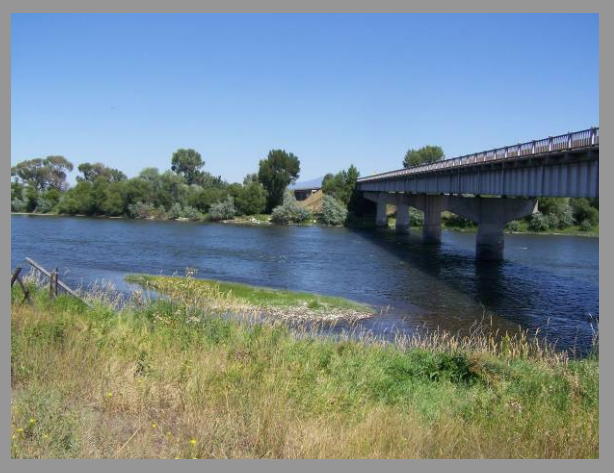
Looking northeast at Missouri River.
