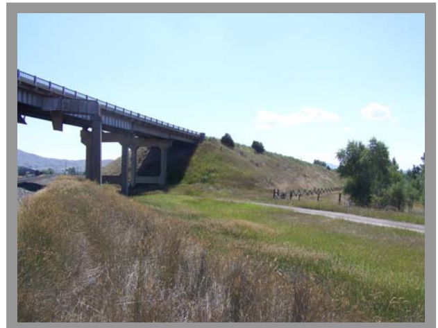
Looking southeast at MRL Bridge and access road.
