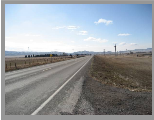
Looking south at US 287.
