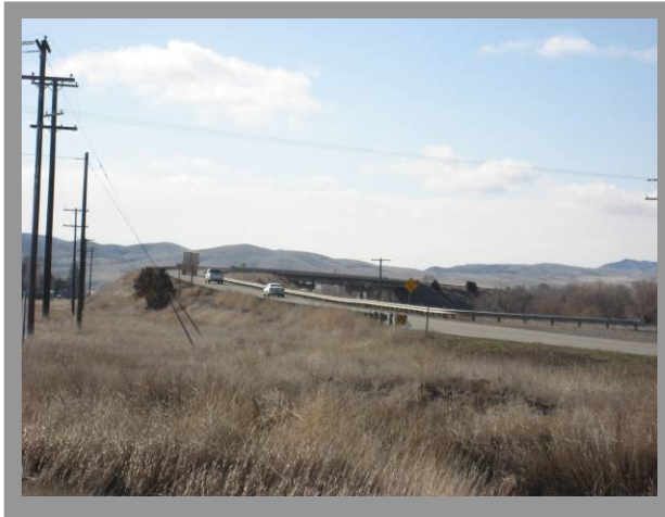
Looking southeast at MRL Bridge crossing.
