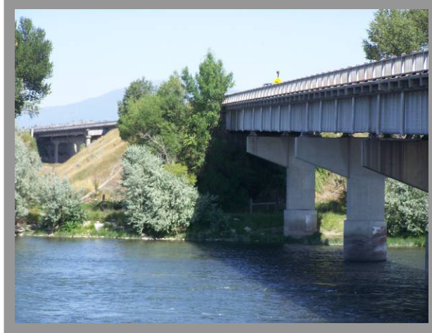
Looking northeast at MRL Bridge and Missouri River Bridge.
