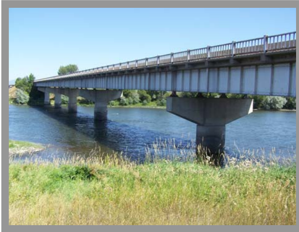
Looking northeast at Missouri River Bridge.
