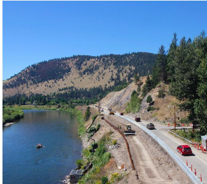
Construction on the erosion wall began with the removal of the old erosion prevention structure. Crews excavated the area and tore out the cement wall that had previously acted as an erosion prevention method.
