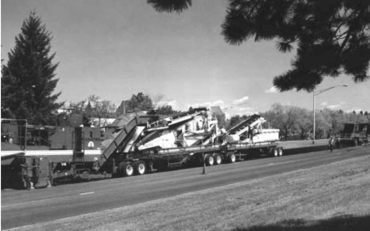
Figure 16-3: Cold In-Place Recycling Arterial City Streets
