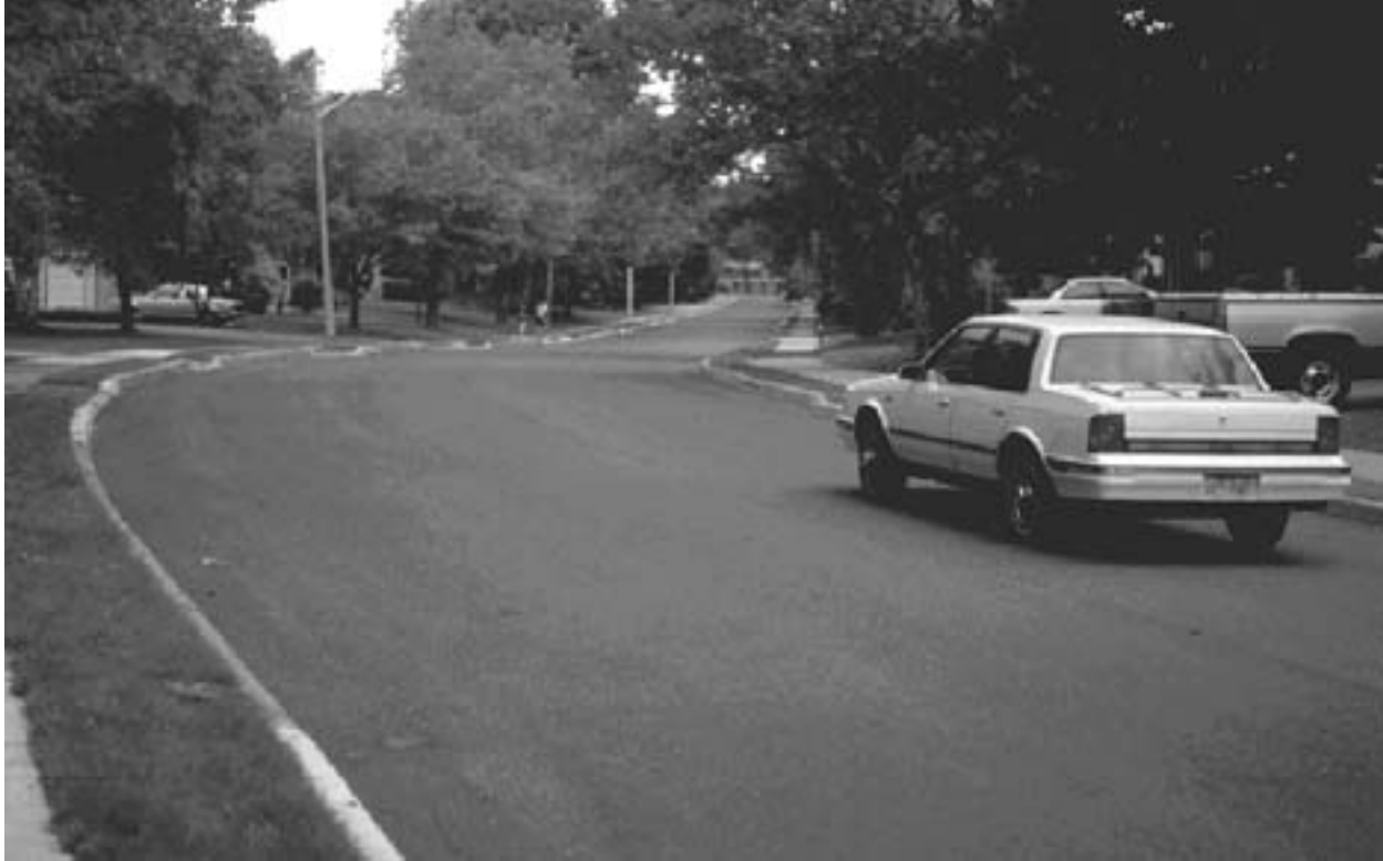
Figure 16-9: Urban Cold In-Place recycled mat prior to placement of wearing surface
