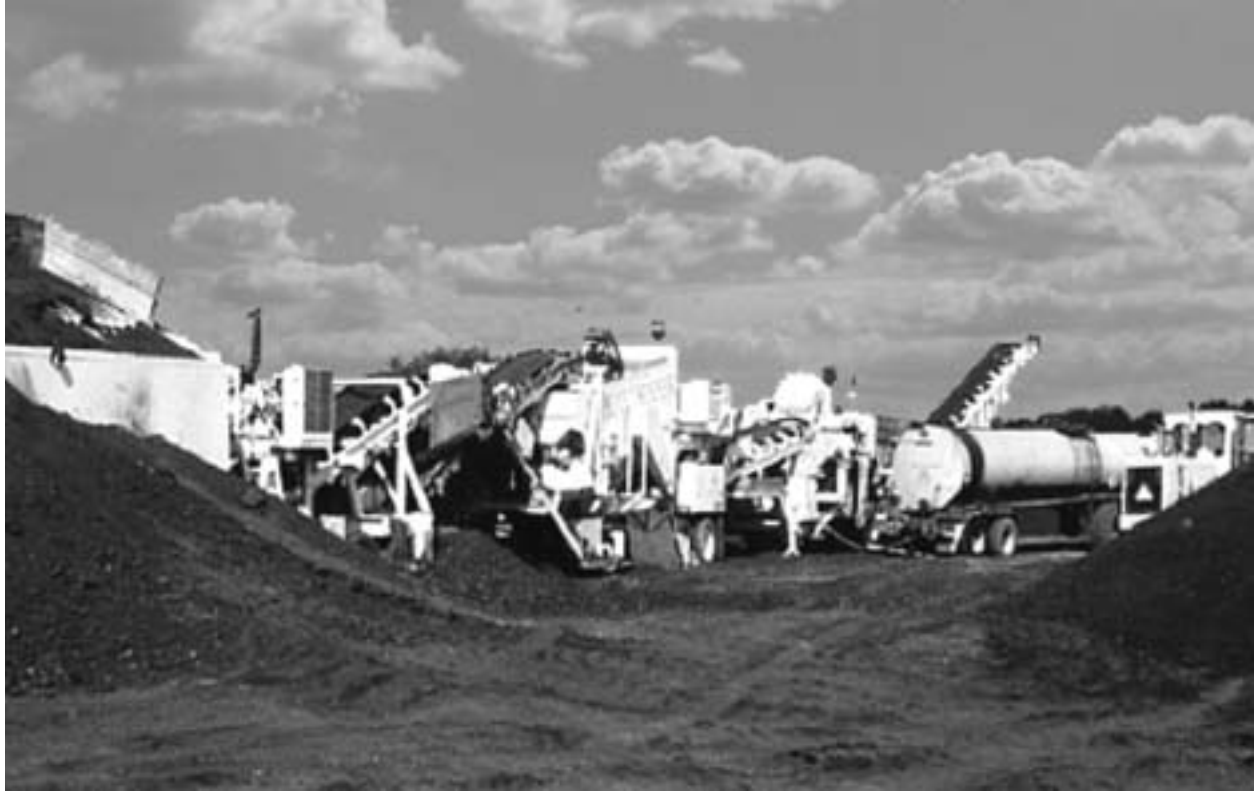
Figure 16-10: CIR Train set up in a stationary plant mode
