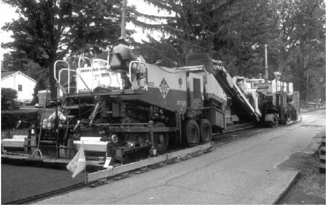
Figure 16-5: Two-unit CIR train
