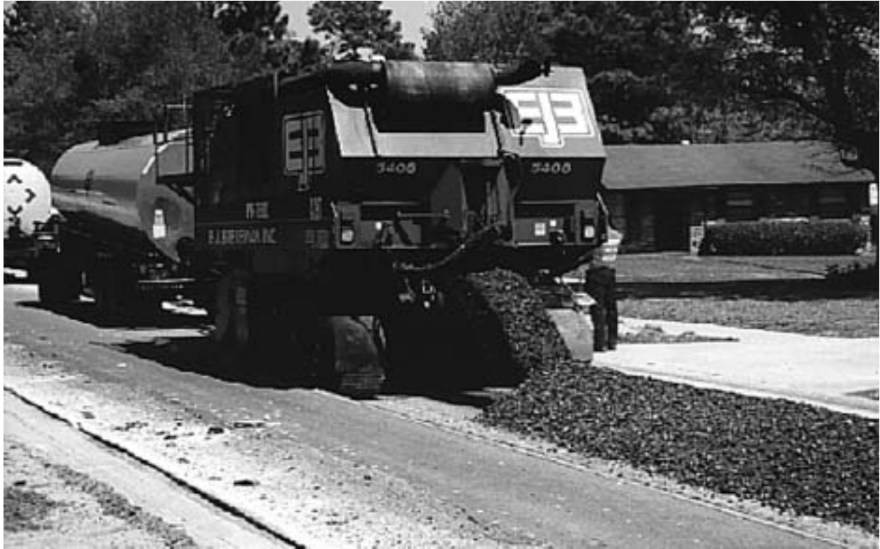
Figure 16-4: Single unit CIR train
