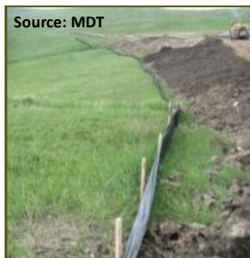
Install silt fence parallel to contours with space for sediment storage.
