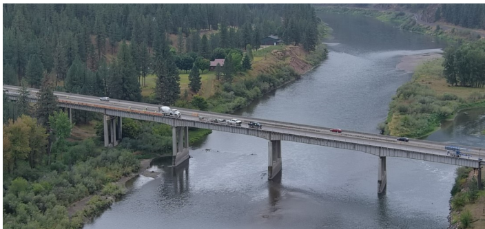
Overhead view of traffic on I 90 bridge near Alberton, Mont.
