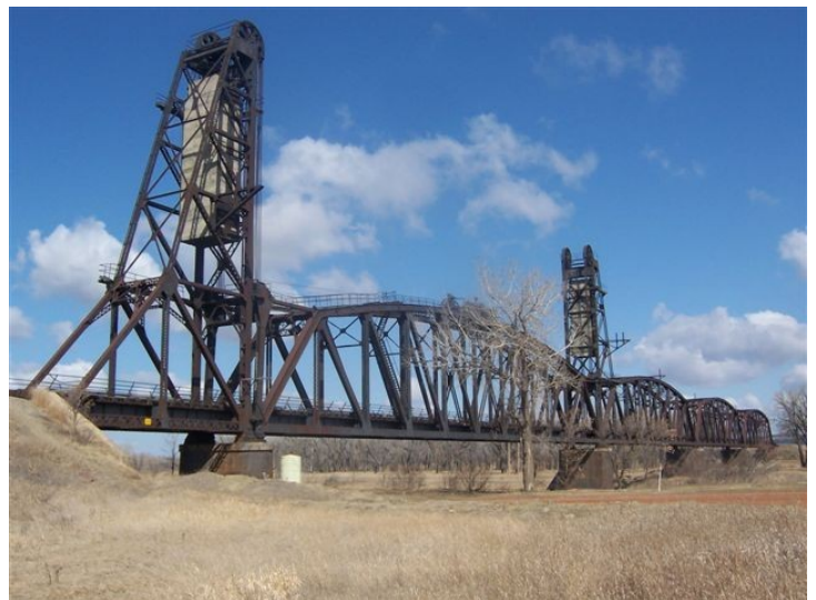
The Snowden Bridge, Montana's only vertical lift structure in the state.
