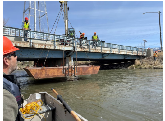
Pictured above: Setting the barge in the Beaverhead River.
