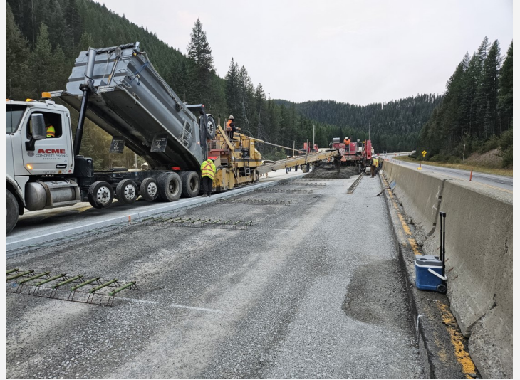
Final passing lane being placed on I 90 in September 2024
