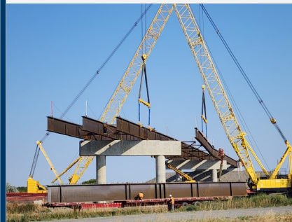
Hanging bridge girders on the Railroad Overpass project segment (pictured left) and the completed Yellowstone River Bridge portion of the Railroad Overpass project segment (pictured below).
