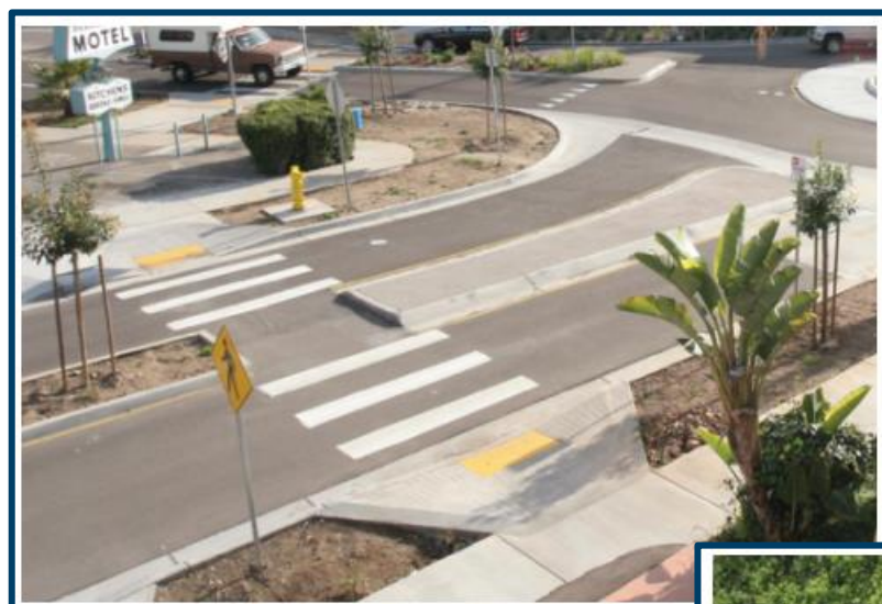
Median and pedestrian refuge island near a roundabout. Source: www.pedbikeimages.org / Dan Burden
