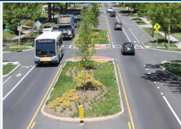
Example of a road with a median and pedestrian refuge islands. Source: City of Charlotte, NC
