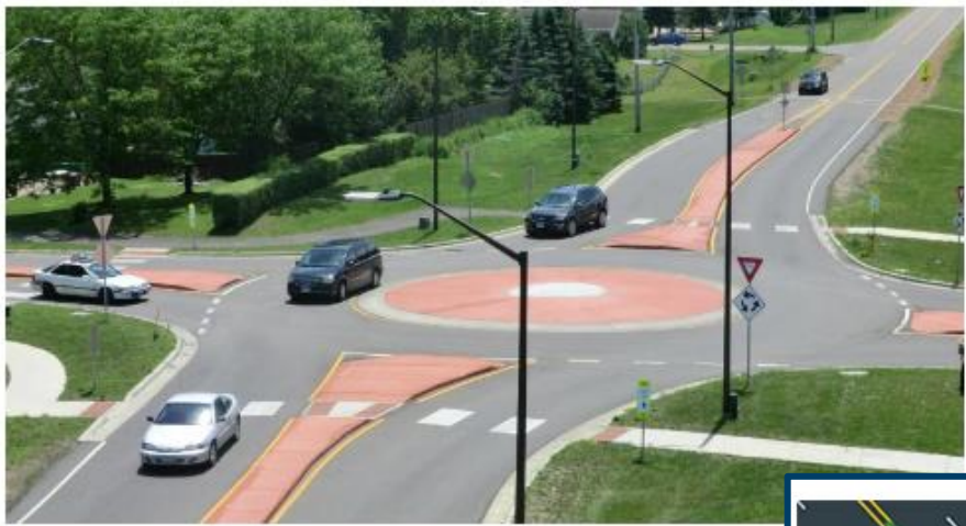
Example of a single-lane roundabout. Source: FHWA
