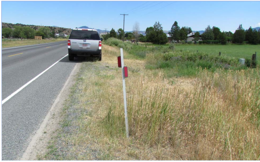
Figure 3- Reflector bent forward
