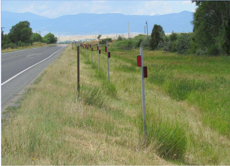
Figure 1- Reflector system cleaned and mowed
