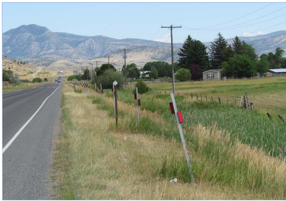
Figure 4- Reflector bent forward
