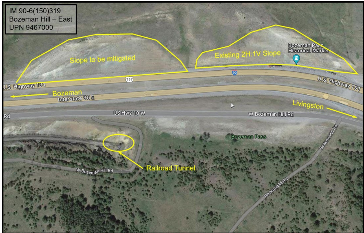
Figure 2: Slope Mitigation Area Aerial Image
