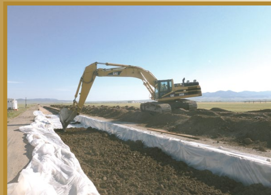
Filling lined trench with subgrade
