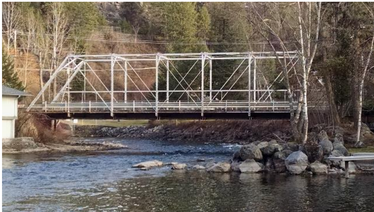
Figure 1: Swan River Bridge in Bigfork
